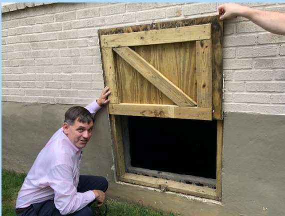
WX staff members examine the crawl space of a clients home during the assessment
